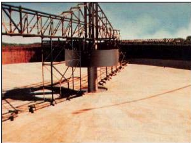
Peripheral Driven Full Diameter Bridge Clarifier
