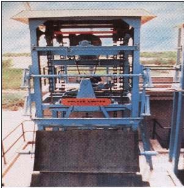
Mechanical Grab Type Screen
