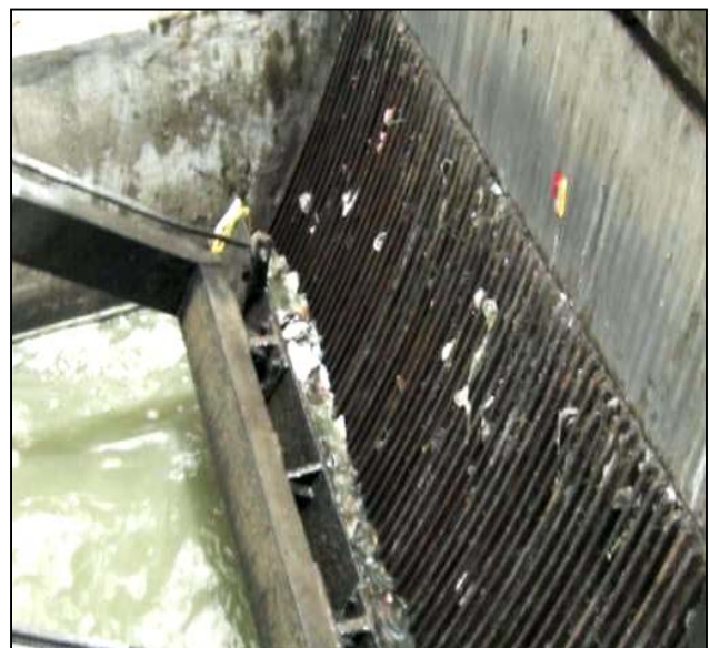
Mechanical Curved Bar Screen
